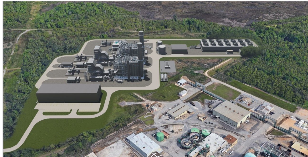
Orange County Advanced Power Station , a 1,215 megawatt facility in Orange, Texas. Construction started in early 2023, and the project is expected to be completed by 2026.
